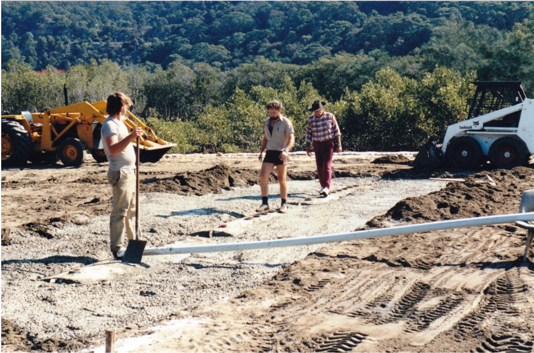
VIEW WEST SOUTH WEST. THREE TANKS IN LINE AND COVERED WITH CONCRETE. SANDBROOK INLET TO THE RIGHT OF PICTURE.
